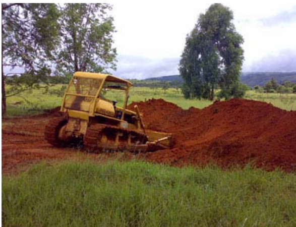
Bulldozer making a water catchment pond
