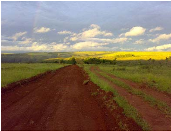
Entrance road, old (on the right) and new
