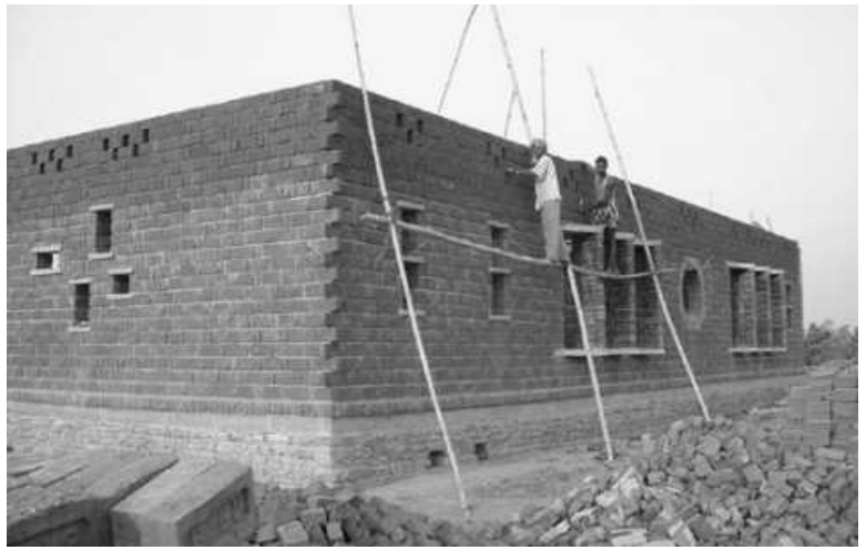
Music College Under Construction
