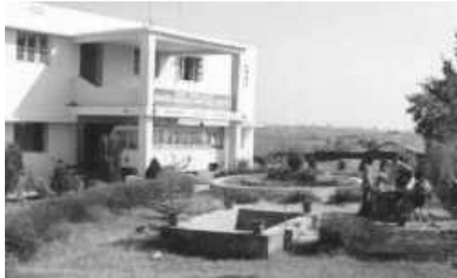
Hospital at Anandanagar
